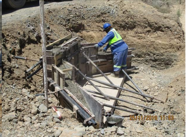
Photo: Casting of concrete on culvert wing wall
