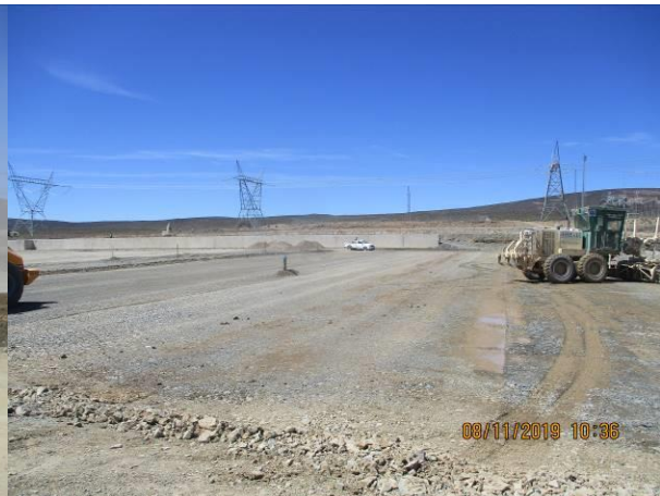
Photo: Final layer works at Section B.
