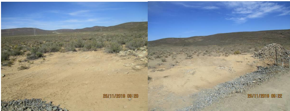
Photos: Damaged area used by excavators during preparation of culverts and V-drain require rehabilitation.
