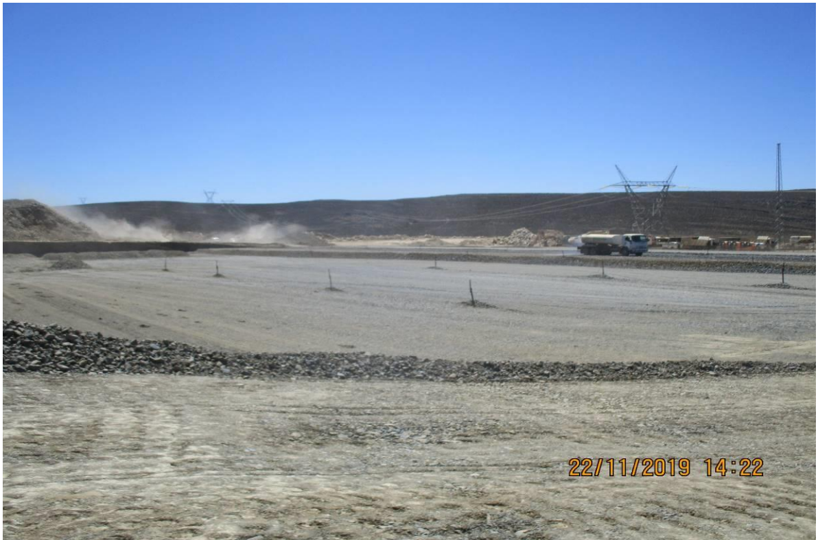
Photo: Layer works in progress at section D.
