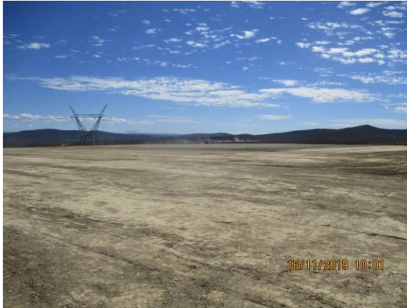
Final layer works at Section A.
