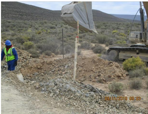
Photos: Culvert wing wall preparations.
