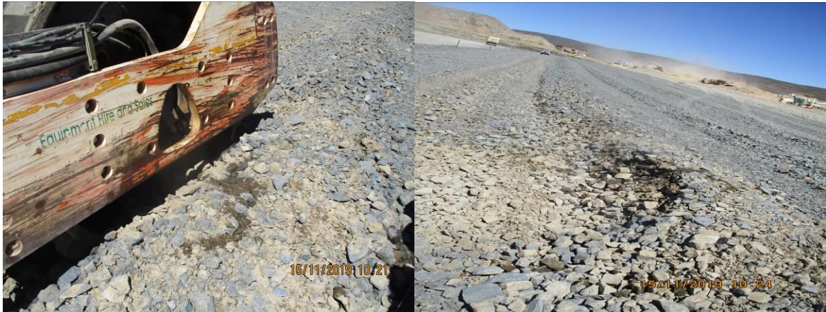
Photo: Hydraulic pipe burst from smooth drum roller.
