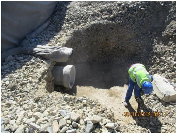
Photo: Preparation of subsoil drainage pipes.
