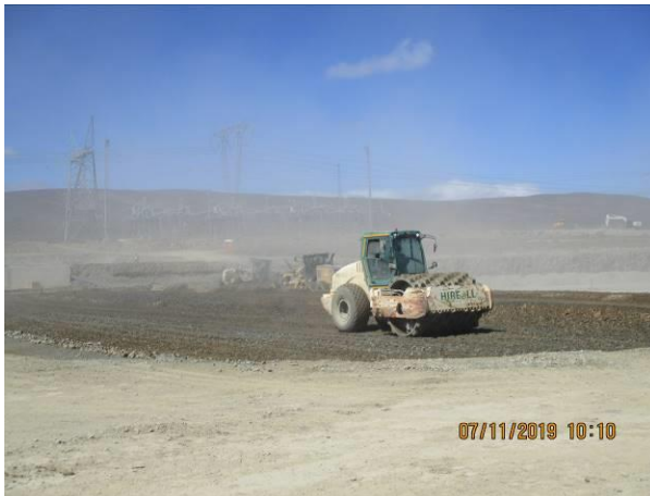
Photo: Layer works at Section B.
