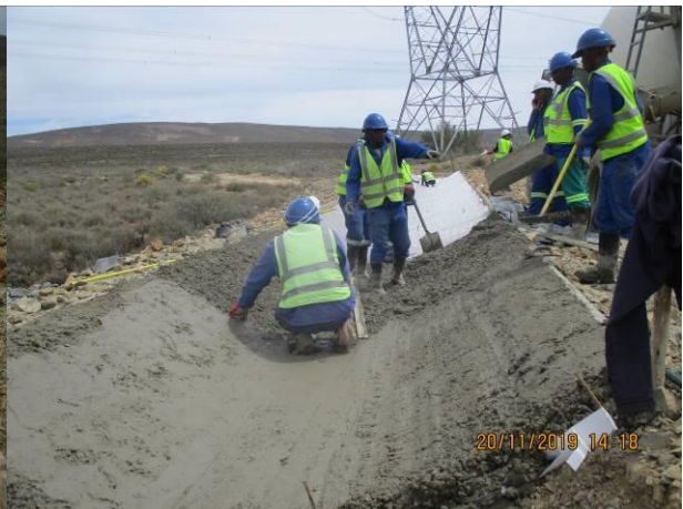
Photo: Casting of concrete on V-drain.
