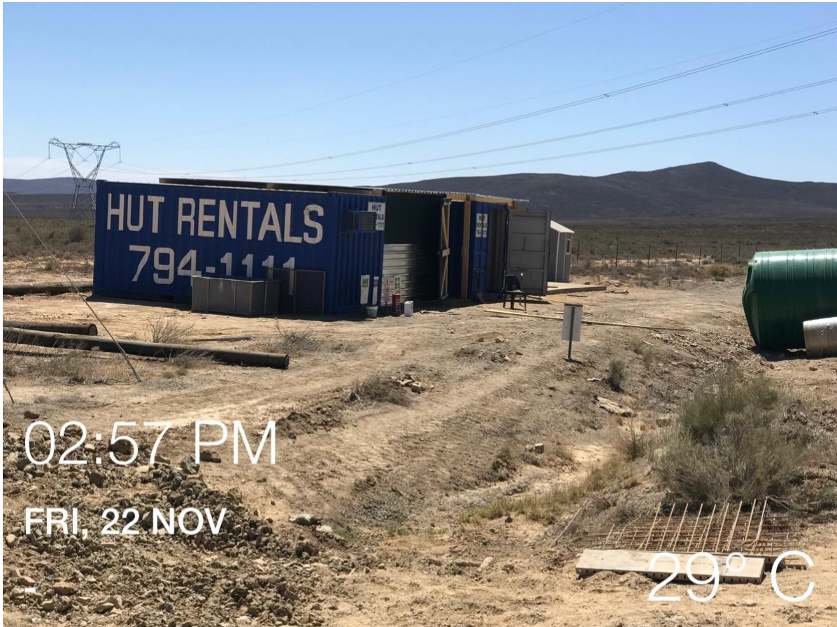
Photo: Site establishment (Civil and building works).
