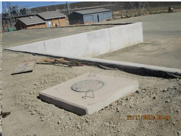
Photo: Mine hall with cover.
