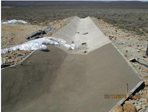
Photo: Final finishing on V-Drain.
