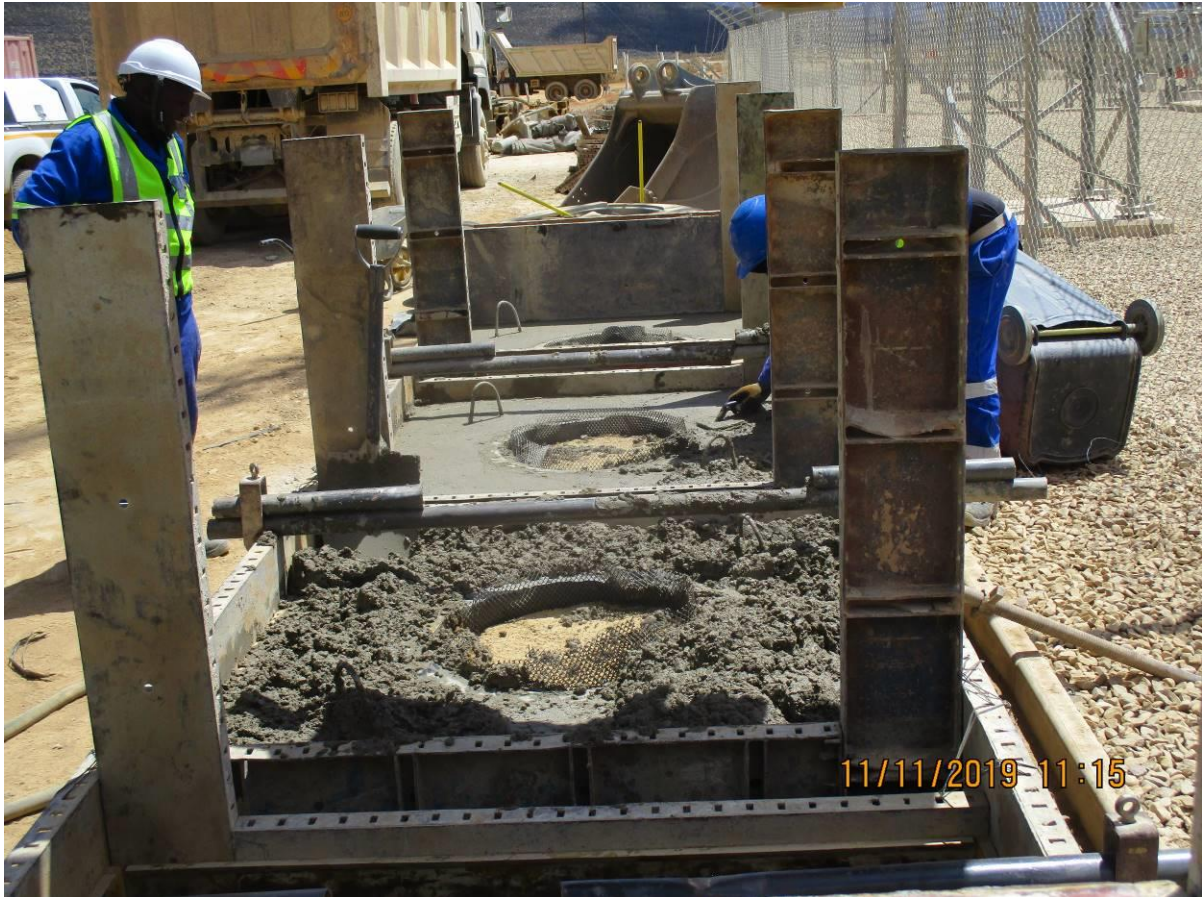
Photo: Casting of mine hall covers.
