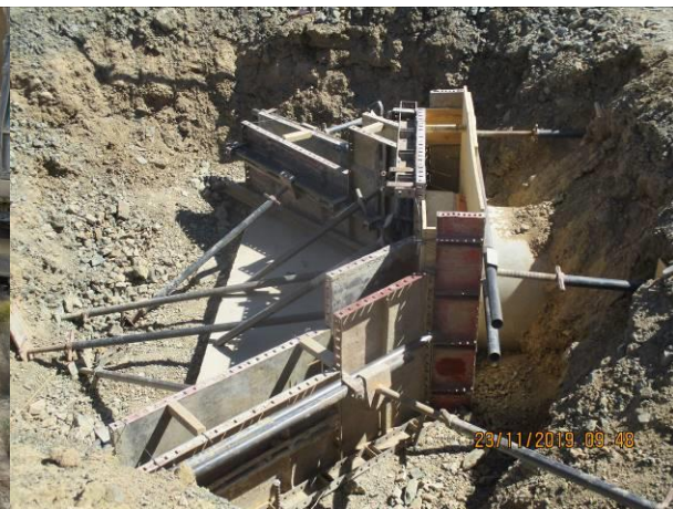
Photo: Casting of concrete on culvert wing wall
