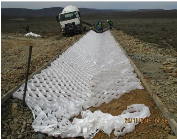
Photo: Geo-cell preparations on V-drain.
