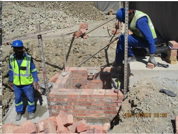
Photo: Construction of mine hall in progress.
