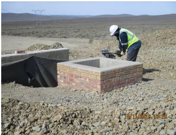
Photo: Mine hall completed.
