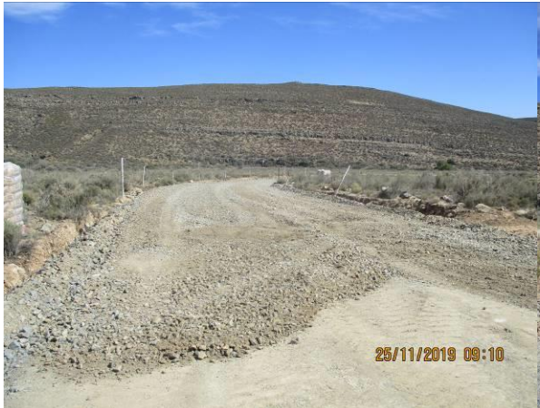
Photo: Final layer on permanent access road.
